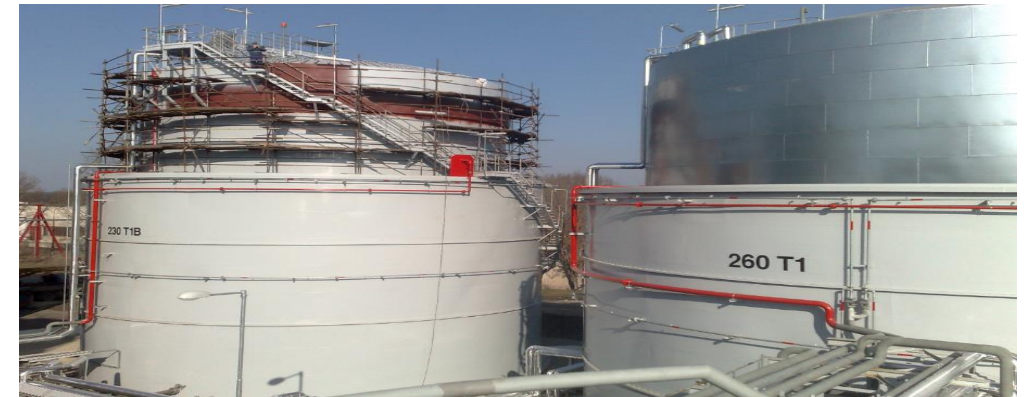
Cylindrical storage tanks for oil, soybean oil
