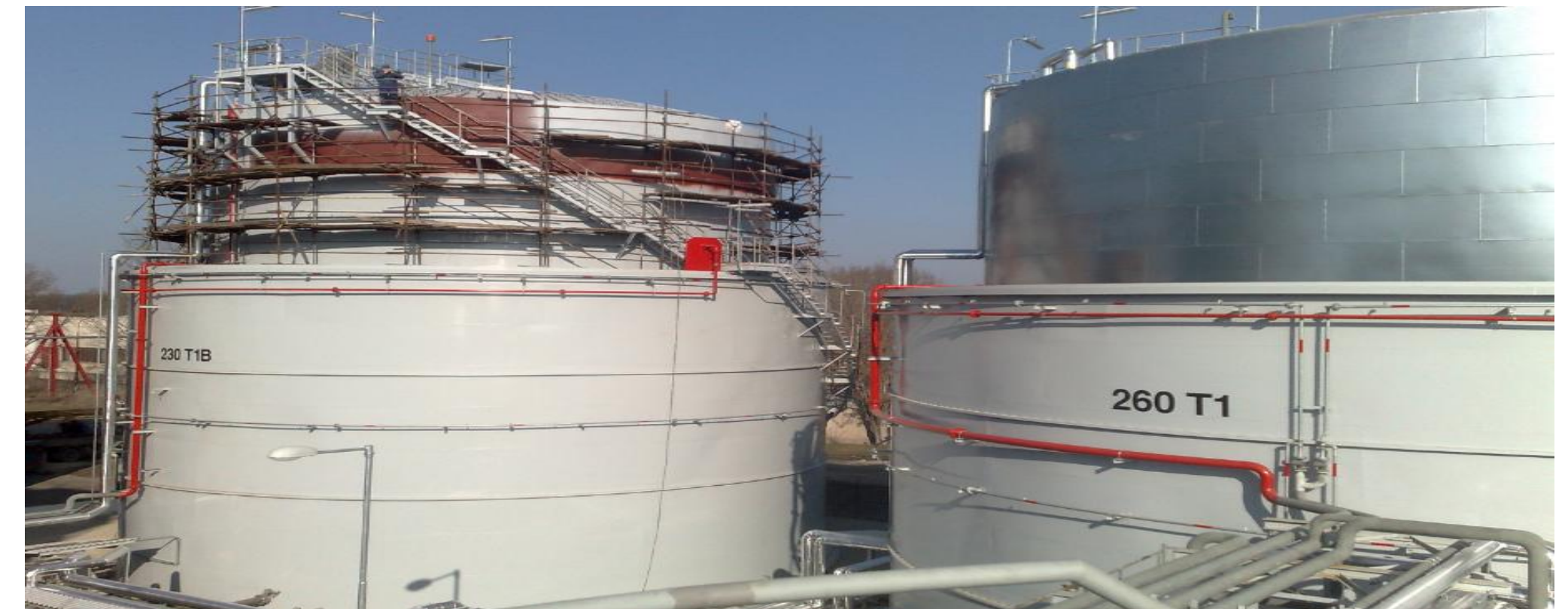
Cylindrical storage tanks for oil, soybean oil
