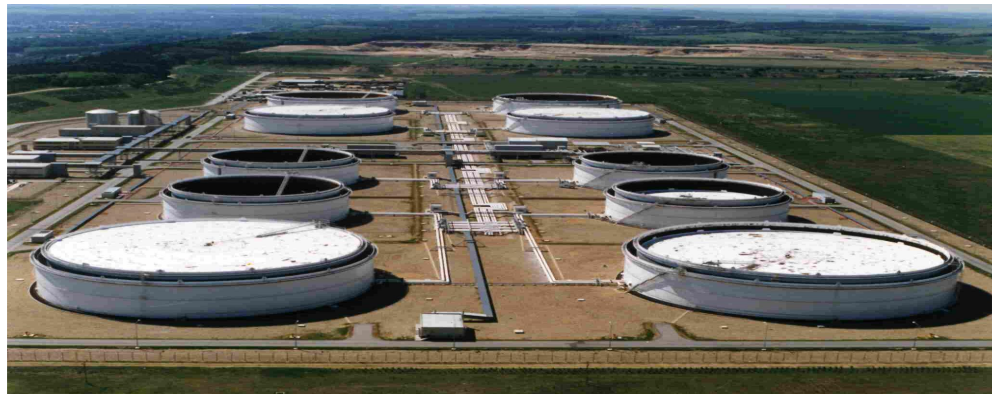
Large-capacity oil tank farm
